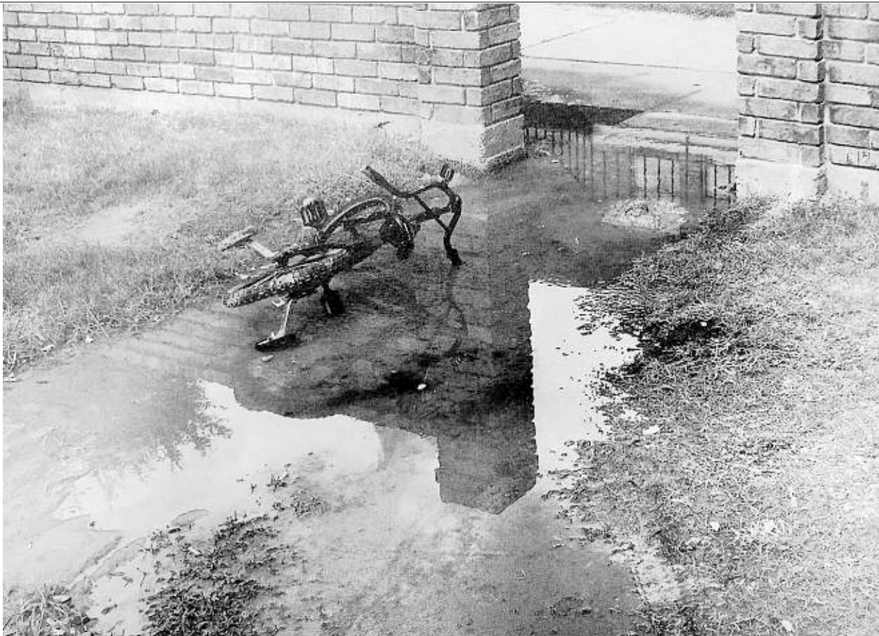
Houston Police Department Environmental Investigations Unit The Yale Court Apartments have had a "long-standing problem with raw sewage," according to police records. A former owner said tenants can be the cause of sewer line problems through ignorance or vandalism.
